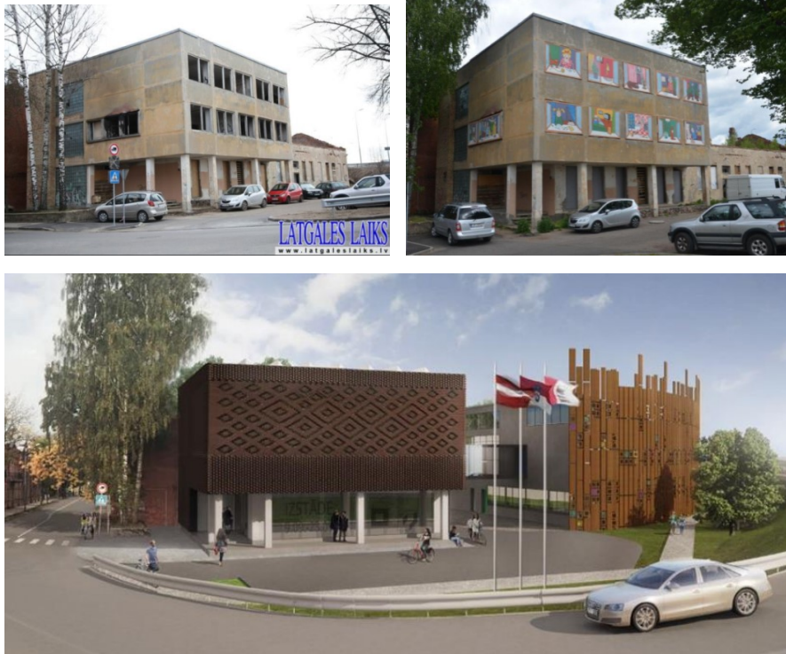
Figure 1 The current state of the building and the project of the new building of "Saules skola" (B1)
