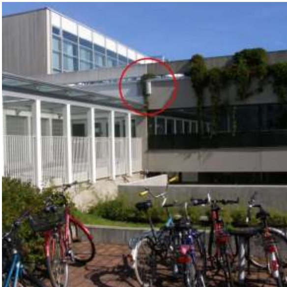
Fig. 1. An example of a mobile communications base station antenna (marked with a red circle), positioned close to ground and building surfaces on top of the entrance; Tampere University campus, Finland.
