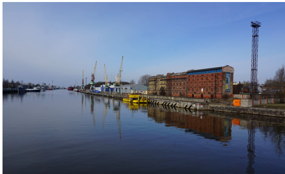
Fig.7. The harmony of the bank building and the Vessels silhouette (photo by authors, 2017.)
