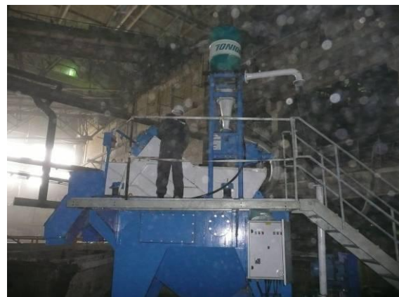
Fig. 10 Fine separation cyclones
