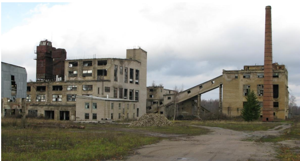
Fig. 1. Former peat factory in Struzani
