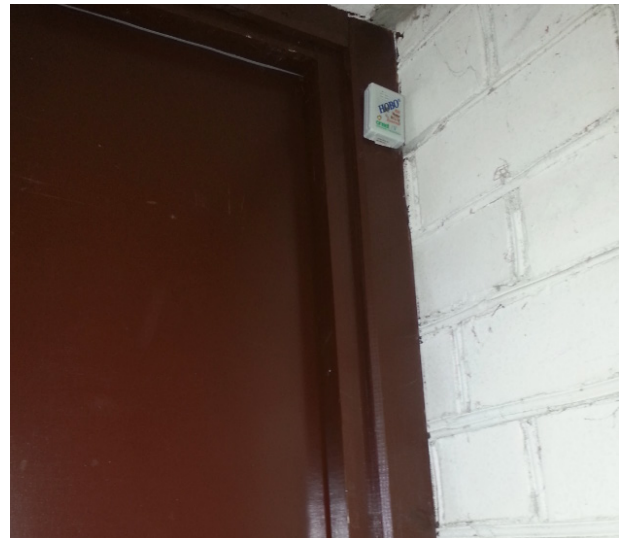
b – inside wooden door
