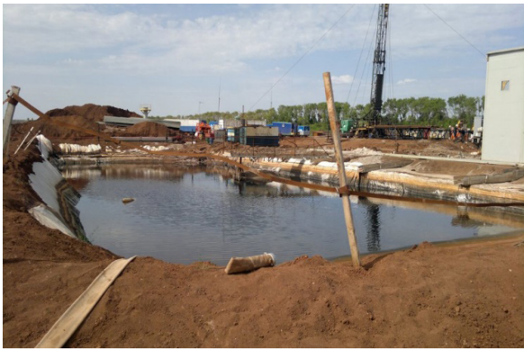
Fig. 1. The two-section mud pit.
