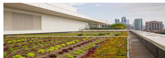
Fig.10. Chicago Botanic Garden's McCormick Place West Rooftop Garden
