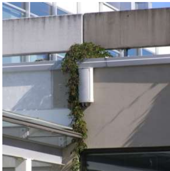
Fig. 2. A close-up of a mobile communications base station antenna, positioned close to ground and building surfaces; Tampere University campus, Finland.
