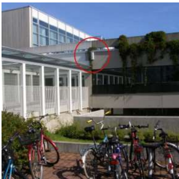
Fig. 1. An example of a mobile communications base station antenna (marked with a red circle), positioned close to ground and building surfaces on top of the entrance; Tampere University campus, Finland.
